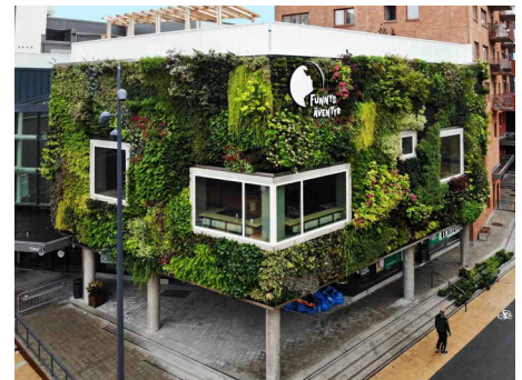
OUTDOOR PLANT WALLS
